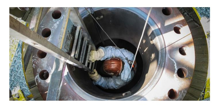
The self-priming, single-coat application of HEGGEL Corr 220 AF not only simplifies the application process but also significantly reduces labor and material costs. This efficiency is especially advantageous for large-scale projects where effective time and resource management are crucial. Additionally, the coating is engineered to cure at ambient temperatures, facilitating a straightforward and energy-efficient application.
